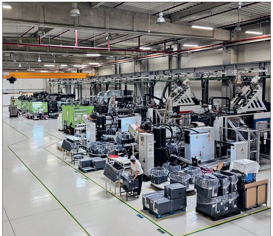
Although the plant is still quite small, it plays a key role in Nolato’s end-to-end offering.
