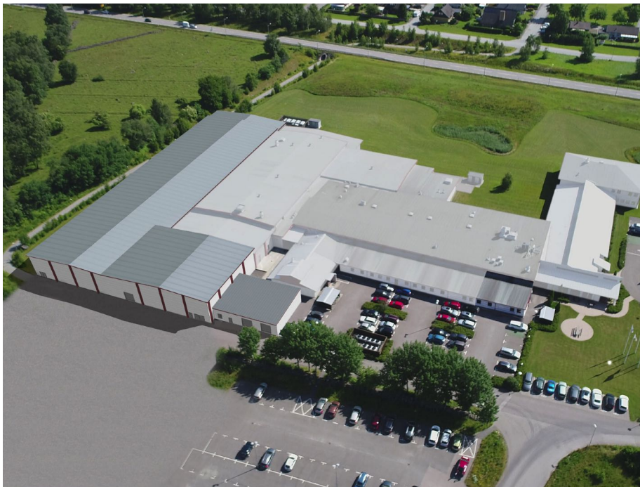
The factory in Hörby is adding new production area of 3,700 sqm (the darker gray parts).
