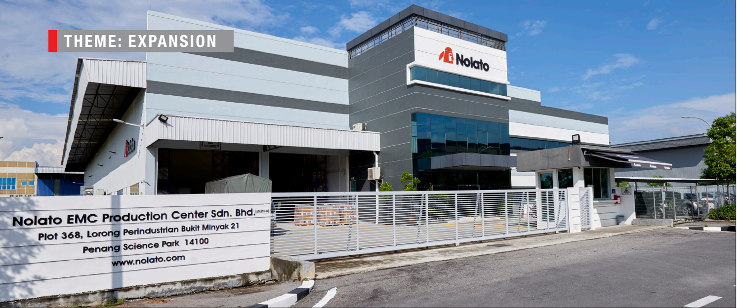
The new Nolato factory in Penang, Malaysia, produces both small design elements for consumer electronics and EMC solutions.
